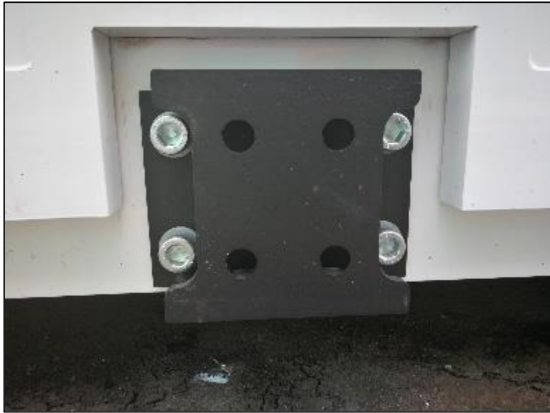
Figure 8 - Crane lifting bracket.
